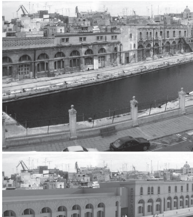
Figure 11 - Dock n° 1 at present and after the recovery
