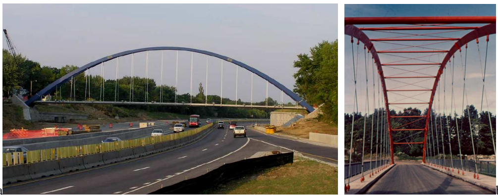
Figure 1. a) Steel tied arch with vertical hangers (Griffin memorial bridge). b) Network arch (Steinkjer bridge)
