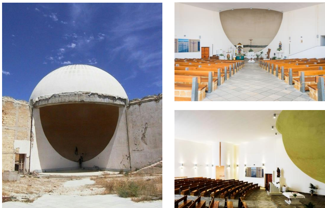
Figure 2. The interiors, before and after the collapse
