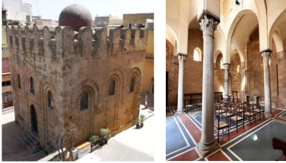
Figure 1: External and internal view of the upper church of San Nicolò Regale.
