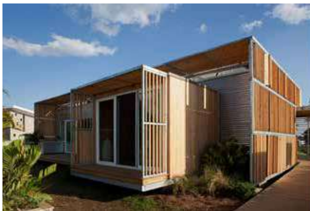
Fig. 3. Flex House @SolarDecathlon
