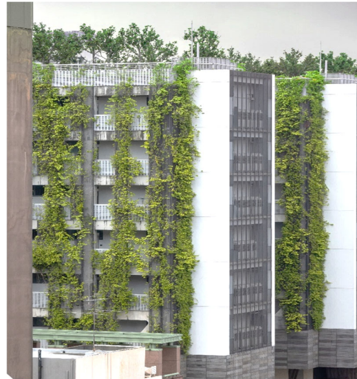
Figure 2. Example of green walls with climbing plants on metal mesh.
