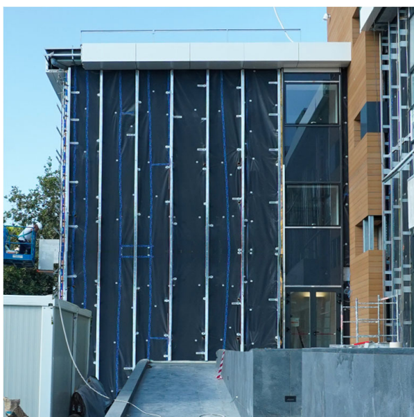
Figure 5. Green Habitat Wall Green Hydro execution phases (Green Habitat srl).
