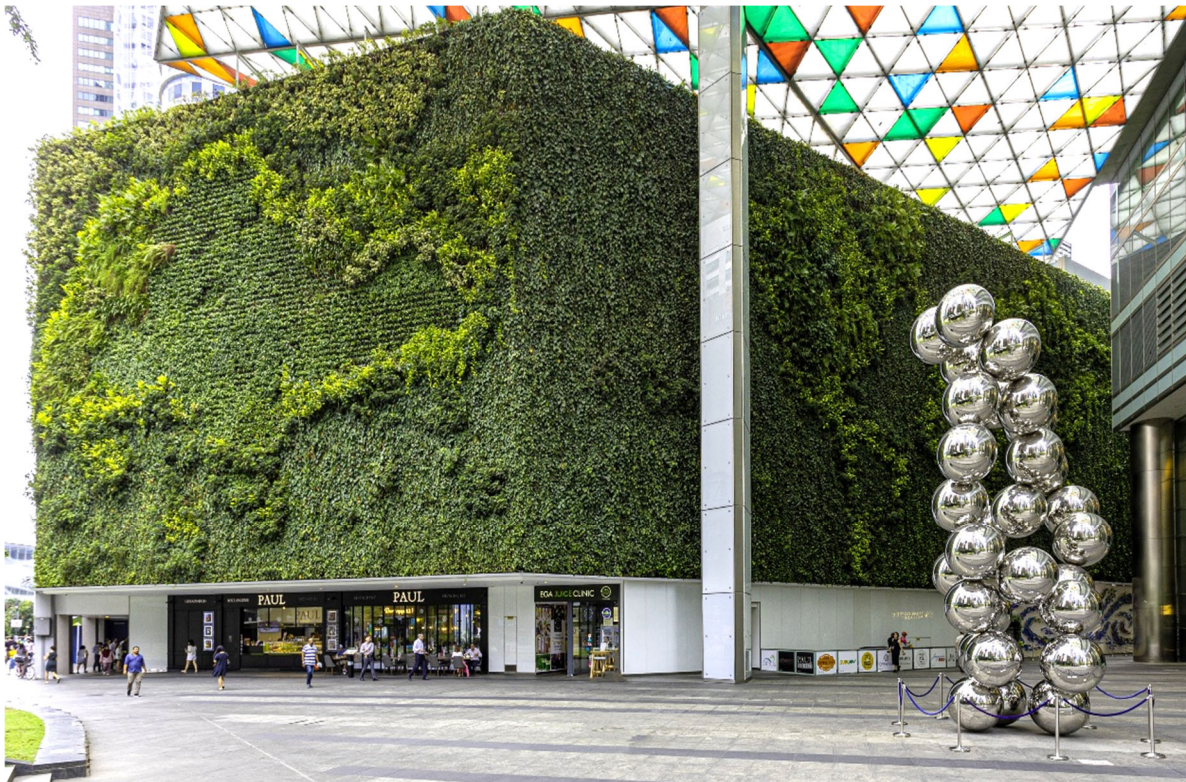
Figure 3. Example of a continuous living wall in Singapore.
