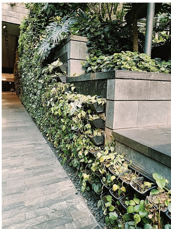
Figure 4. Example of a modular living wall with pots.
