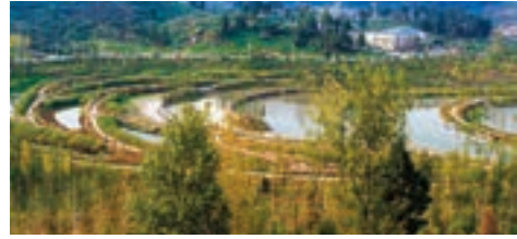
Fig. 4 | The new Shuicheng river terraces, Liupanshui Minghu Wetland Park, designed by Turenscape (credit: Turenscape, 2013).
