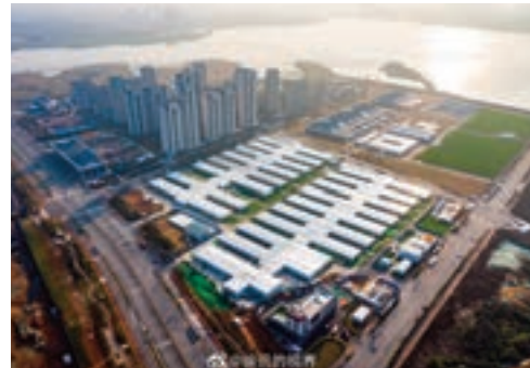
Fig. 11 | Global view of off-site modular units in the Wuhan Leishenshan Hospital project (source: archdaily.com).
