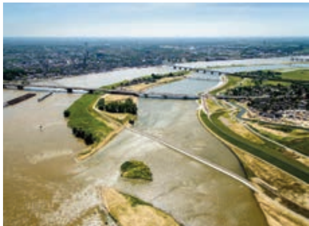
Fig. 7 | New cycle/pedestrian crossing and new wetland ecosystems on the side of the I-Lent Riverpark Nijmegen, designed by Lodewijk van Nieuwenhuijze and H+N+S landscape architects (credit: COAC, 2016).
