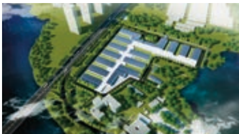
Fig. 8, 9 | Wuhan Huoshenshan Hospital is the world's first large-scale temporary facility built in record time to accommodate people infected with Covid-19. Designed in 24 hours with BIM methodology and created by CITIC Architectural Design Institute and China Construction Third Engineering Bureau, by a team of approximately one thousand five hundred workers and five hundred construction machines, at the request of the Wuhan municipal construction unit (source: redshift.autodesk.it; credit: CITIC ADI).
