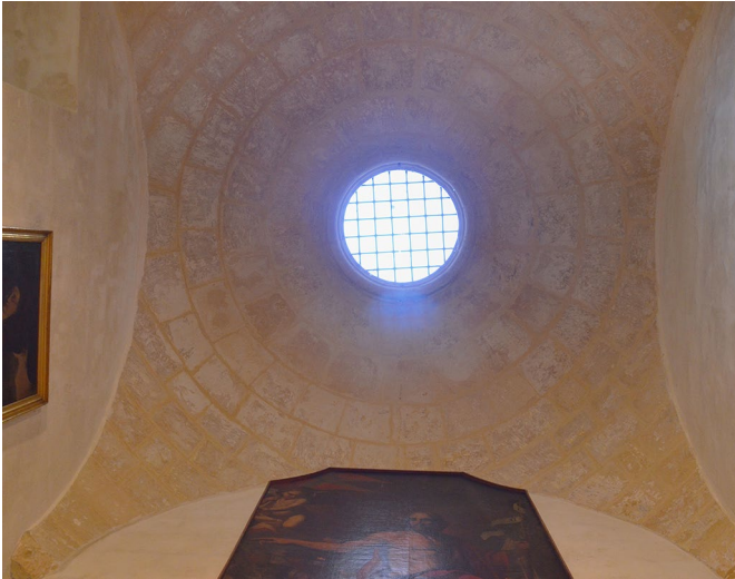
Fig. 10 La Valletta, sail vault over the sacristy in the church of St. Barbara
