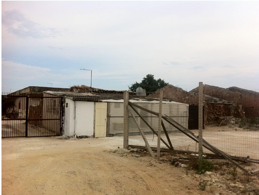
Fig. 4 Example of a structure adapted for housing by migrants in the province of Ragusa (Sicily). (Photos by Todaro V)
