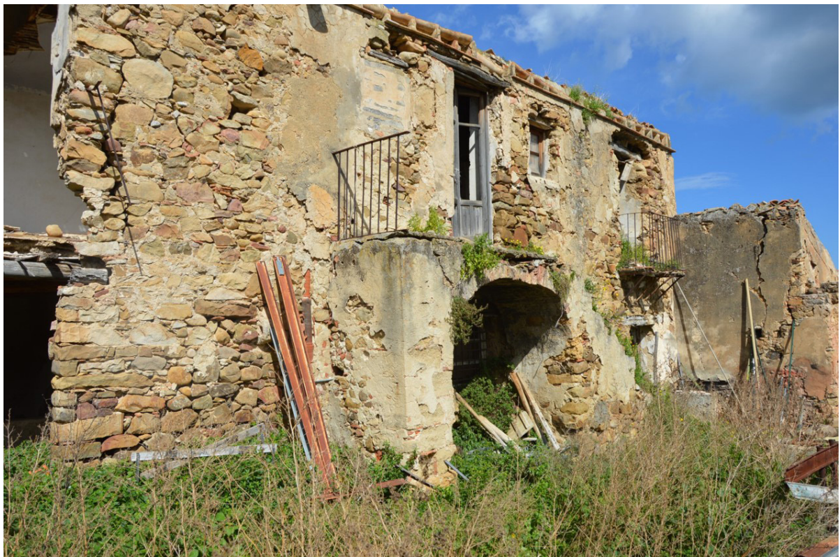
Fig. 6. Example of rural architecture in Sicily, object of a necessary and compatible rehabilitation intervention (photo by the author).
