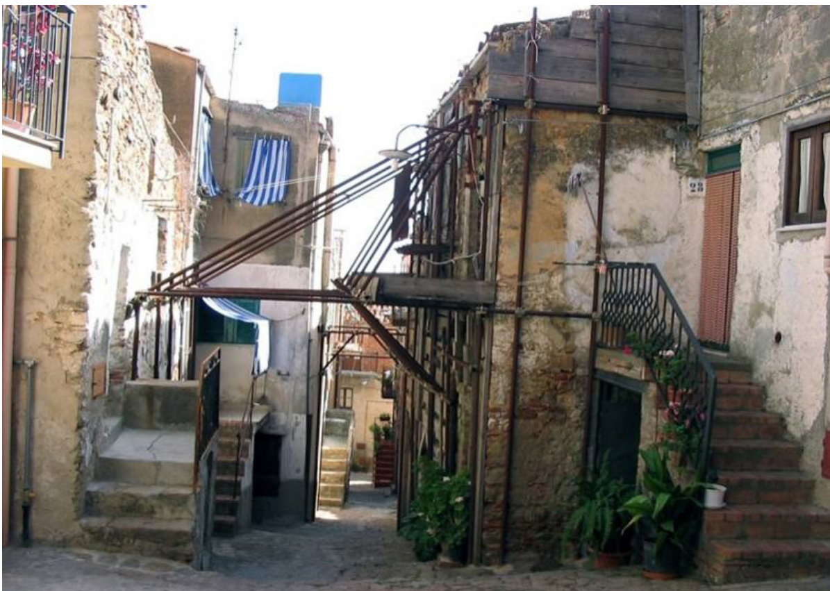
Fig. 4. Detail of the state of abandonment of traditional architecture inside the Madonie inner area (photo by S. Lo Piccolo)..
