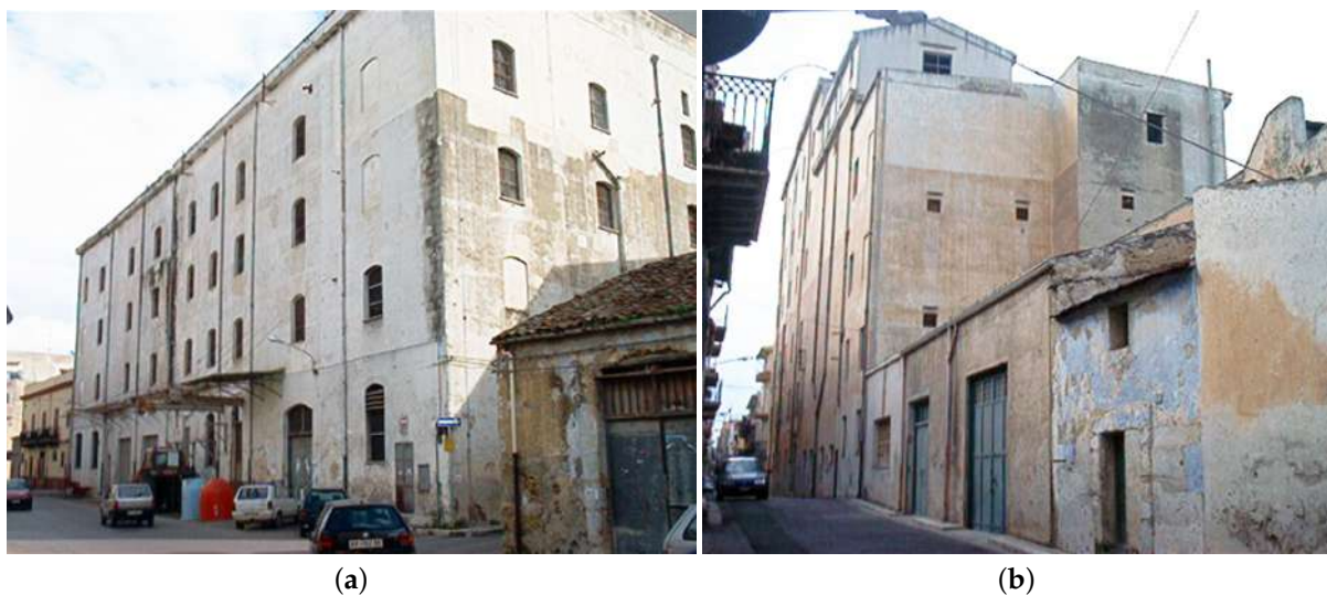
Figure 7. Building exterior views. (a) Main front; (b) Secondary front.
