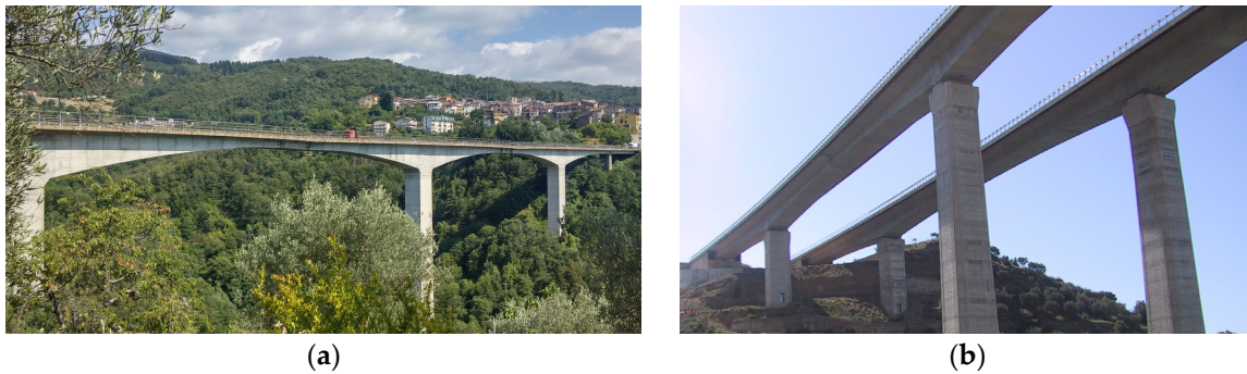
Figure 1. (a) Cannavino bridge on the roadway between Paola and Cosenza, Italy, with clamped deck on piers and drop-in span; (b) Bridge on the A20 motorway in Sicily, Italy, with continuous box girder on piers.
