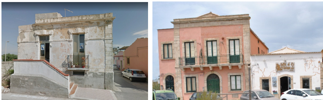
Figure 2: Typical masonry buildings in Marzamemi.
