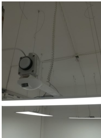
Figure 16. Sensors and luminaires installed in Lampedusa.
