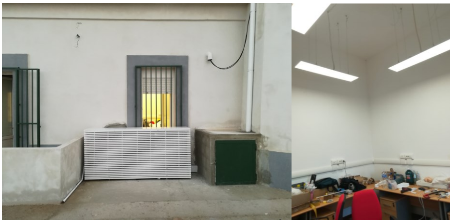
Figure 12. The external (left) and internal (right) views of the room.
