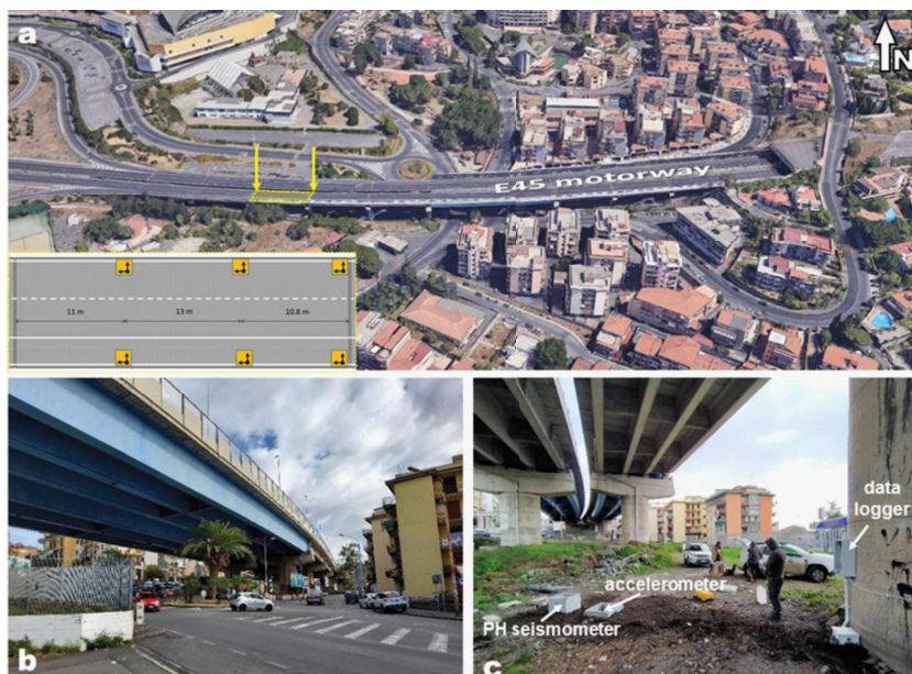
Fig. 1 - a: Google Earth view of S. Paolo bridge (the arrows indicated the segment under investigation) and plan view of sensors location for the experiments; b: lateral view (southern flank) of the structure; c: location of the posthole (50 m deep) seismometer and ground-level accelerometer.
