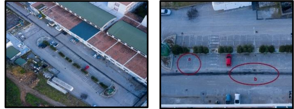
Figure 1 View from the top of the road within the University of Palermo Campus on the left; Selected pavement distresses for ground truth 3D models: potholes a), rutting b).
