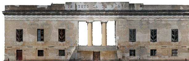
Figure 8. Orthophoto of South-West façade.
