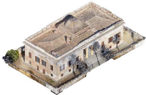
Figure 6. Point cloud of the external parts of Villa Castelnuovo.
