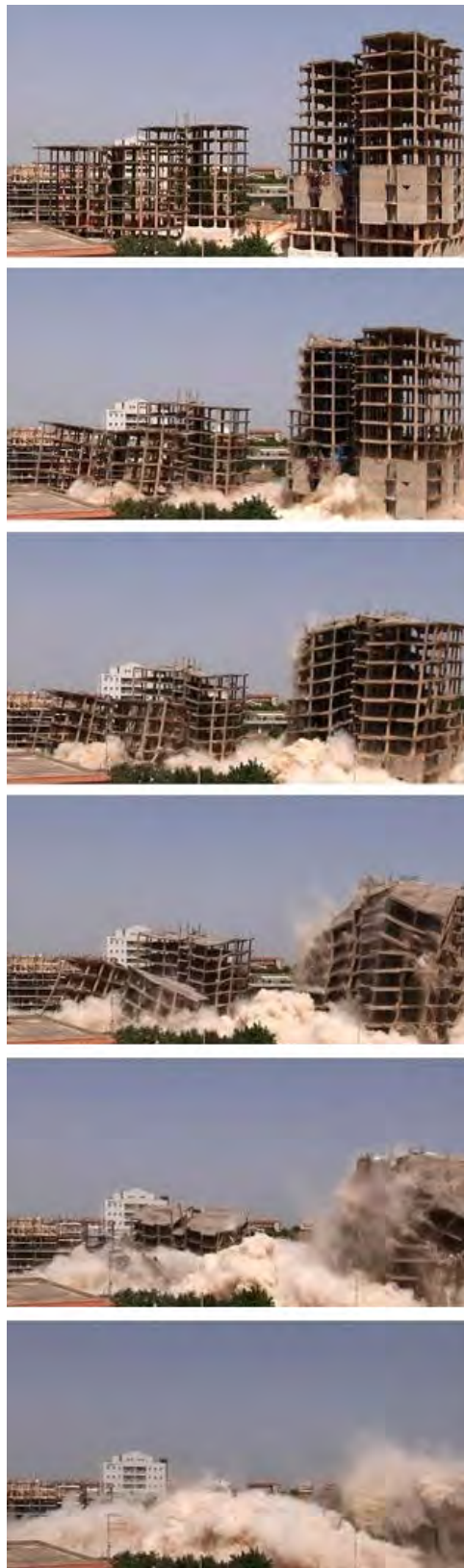
Fig. 37 | Still video da "Demolition#1 squatter" (credit: Loredana Longo)
