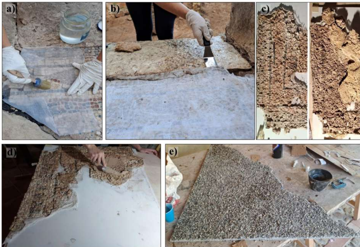
Figure 16. The archaeological restoration: (a) Coating with cotton gauze to carry out the removal of the fragment; (b) Detaching of tessellatum; (c) Mechanical removal of the deteriorated mortar; (d) Application of a new hydraulic mortar; (e) Relocation of the mosaic on new support.
