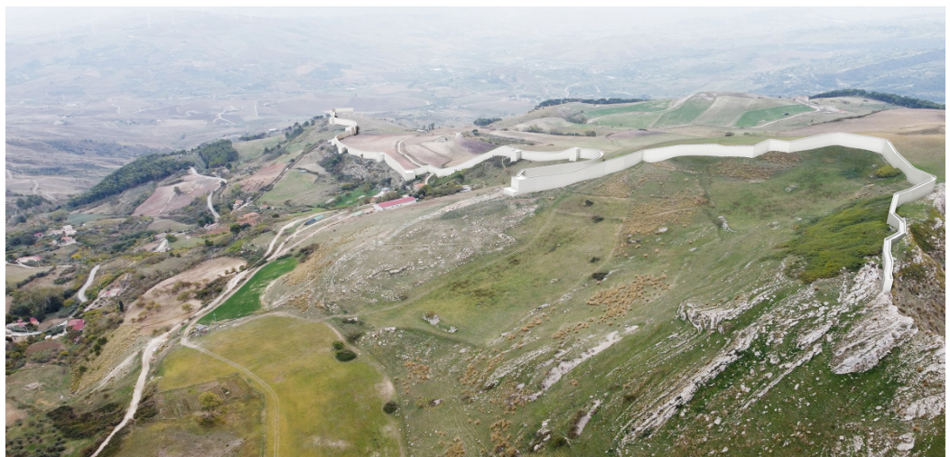
Fig. 7. Photograph taken from a drone with the reconstruction model of the walls inserted. On the right, the highest part of the fortification; on the left and in the background, the Platani River Valley.
