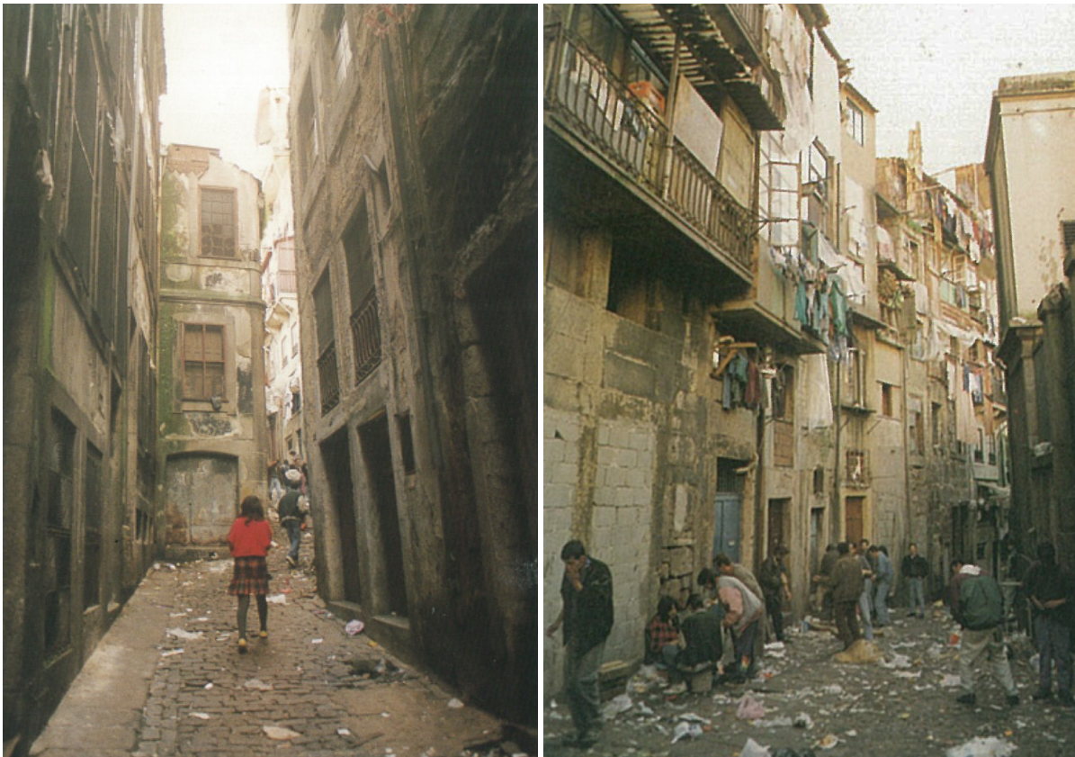
Fig. 4. Critical physical and social situation in Bairro da Sé do Porto in late 1980s. Drug abuse combined with unsafe physical state of conservation of the built environment [Câmara Municipal do Porto, 1998].
