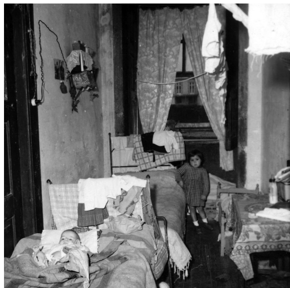
Fig. 2. Inside of a substandard dwelling in th historic centre of Porto, late 1960s (Porto, Arquivo Municipal do Porto).
