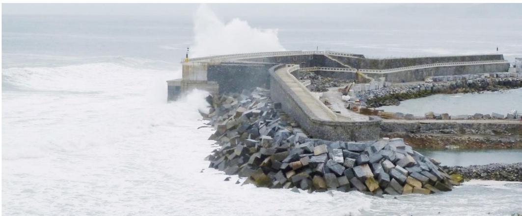
**Figure 18. OWC plant installed in the bay of Mutriku (Spain)**
