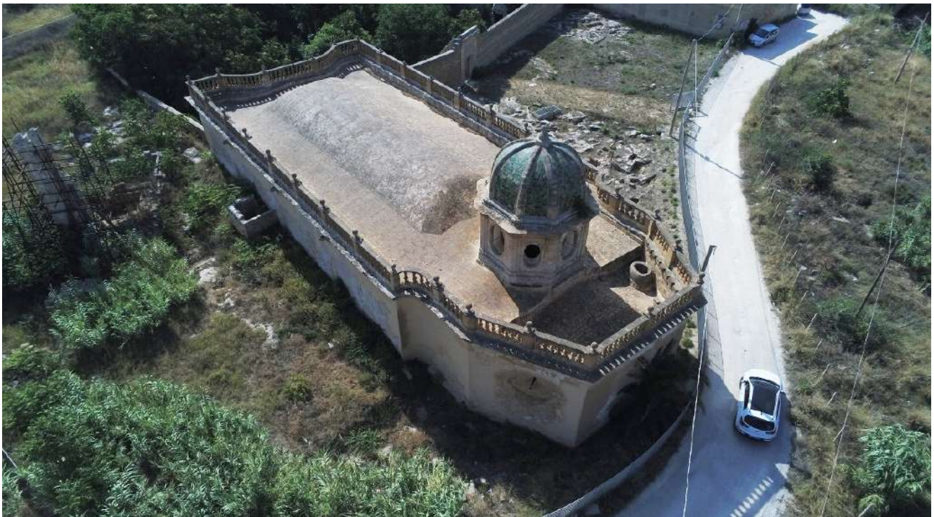
Figure 4. The green tile hemispherical dome of the church of “Santa Maria della Grotta”.
