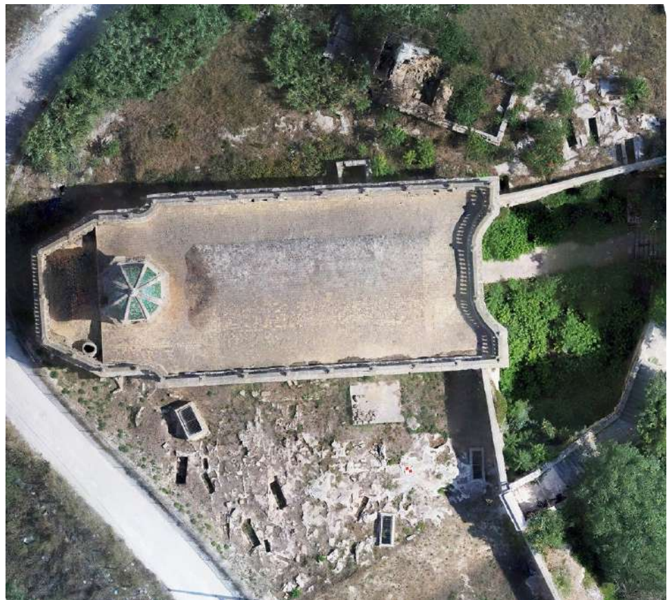
Figure 2. Nadir picture of the “Santa Maria della Grotta” site and building.
