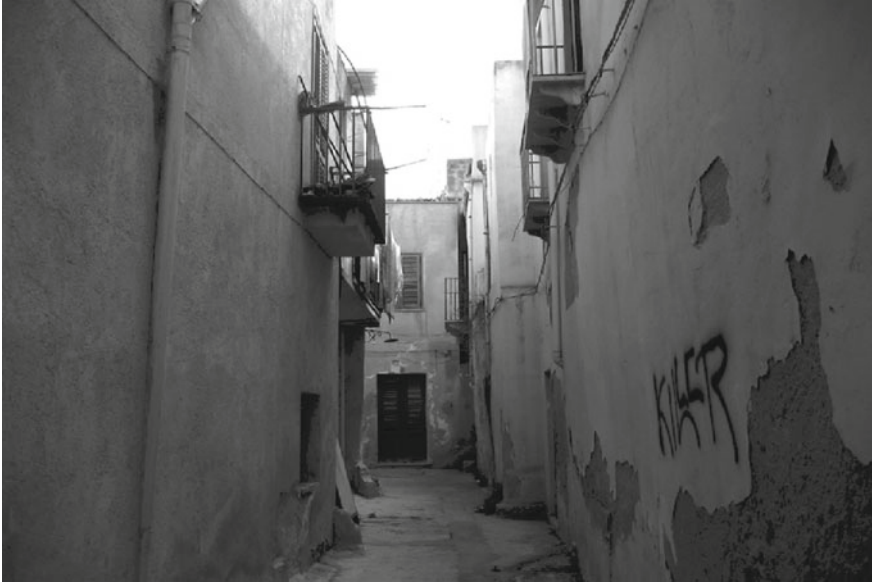
Fig. 2 The deterioration of the part of the historic centre that is inhabited by the Maghrebian community (Photo by Vinci I)
