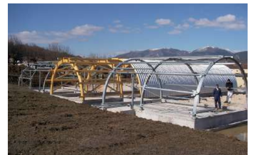
Fig.5 – Construction of the building's structure
