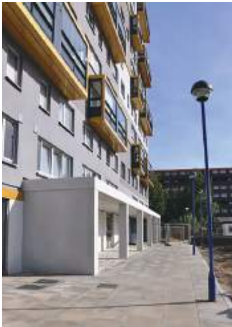
Fig. 4 | Woodside Multi Storey Flats after the retrofit, by Collective Architecture, Glasgow (credit: Collective Architecture, 2019).
