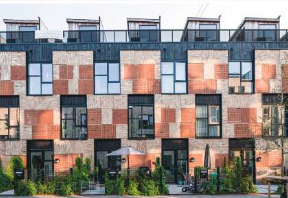
Fig. 1 | The Resource Rows housing complex in Ørestad (DK), designed by Lendager Arkitekter (2015-2019), features reused wall facings on the building envelope; these were cut from the walls of an unused industrial building and consist of prefabricated, framed, multilayer panels (credit: Lendager Arkitekter, 2019).
