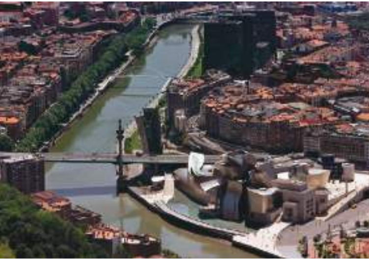
Fig. 7 | Guggenheim Museum by Frank O. Gehry, Bilbao, 1997 (source: guggenheim-bilbao.eus).
