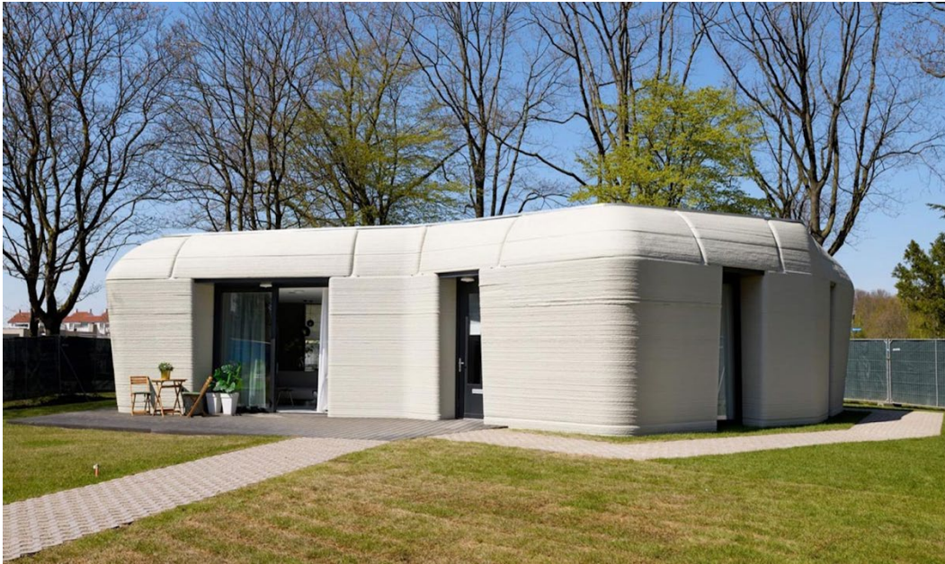
Fig. 11. Eindhoven: A 3D-Printed Concrete House within the Project Milestone Framework
