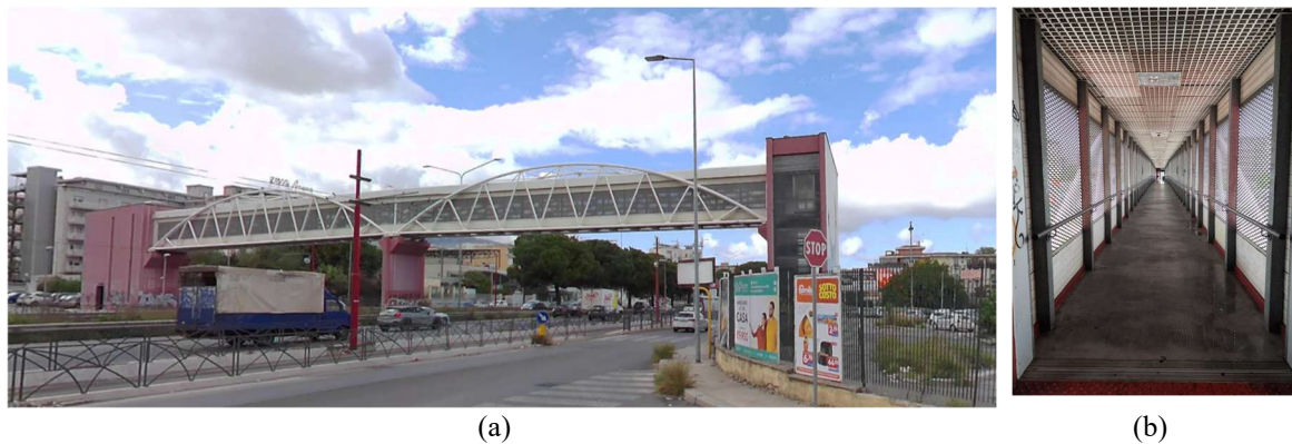
Fig.3. Via Emiri pedestrian footbridge in Palermo: (a) external view; (b) internal view.
