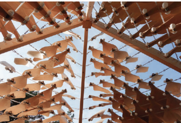
Fig. 2 | Shiver House designed by NEON: a kinetic 'animal like' structure which moves and adapts in response to surrounding natural forces, Korppoo, Finland, 2019 (credits: www.neon.uk/?utm_medium=website&utm_source=archdaily.com/#shiver-house/ ).
