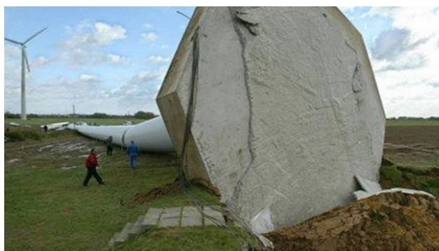
Fig. 2 Catastrophic failure of a wind tower
