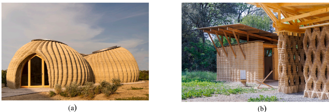
Fig. 1. 3D printed soil structures (a) TECLA (Italy) [31] (b) Earth Forest campus (Spain) [32].
