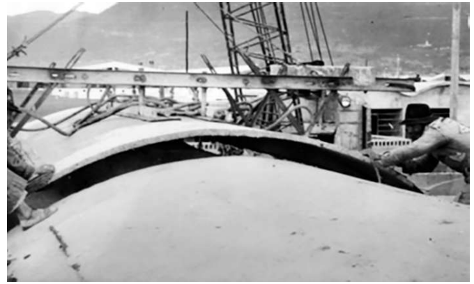
Fig. 6. Left: construction of the shells above a wooden formwork with vacuum concrete. Right: setting a shell as a roofing for a residential unit through the Vacuum Lifter method. Source: [29].
