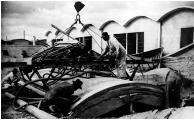
Fig. 6. Left: construction of the shells above a wooden formwork with vacuum concrete. Right: setting a shell as a roofing for a residential unit through the Vacuum Lifter method. Source: [29].
