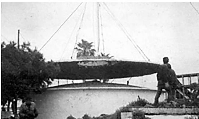
Fig. 5. Top left: transportation of two of the arsenal vaults. Top right: structural section showing vault reinforcing bars and steel reinforced mesh. Bottom left: lifting the dome from the tank used as formwork. Bottom right: structural section of the dome. Source: [27].
