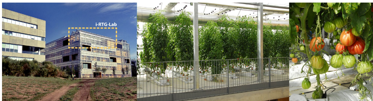
Fig. 1 ICT-ICP building (left), inside of the i-RTG-Lab (middle) and experimental tomato crop (right)
