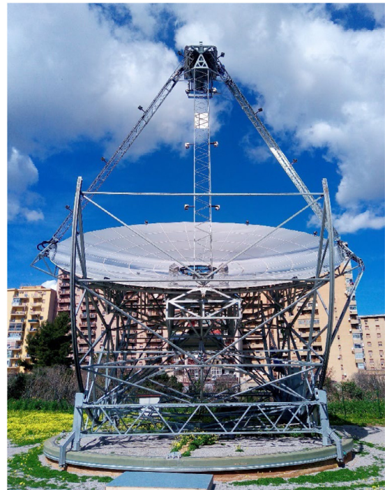
Fig. 3. The dish-Stirling CSP plant installed at the university campus in Palermo (Italy).
