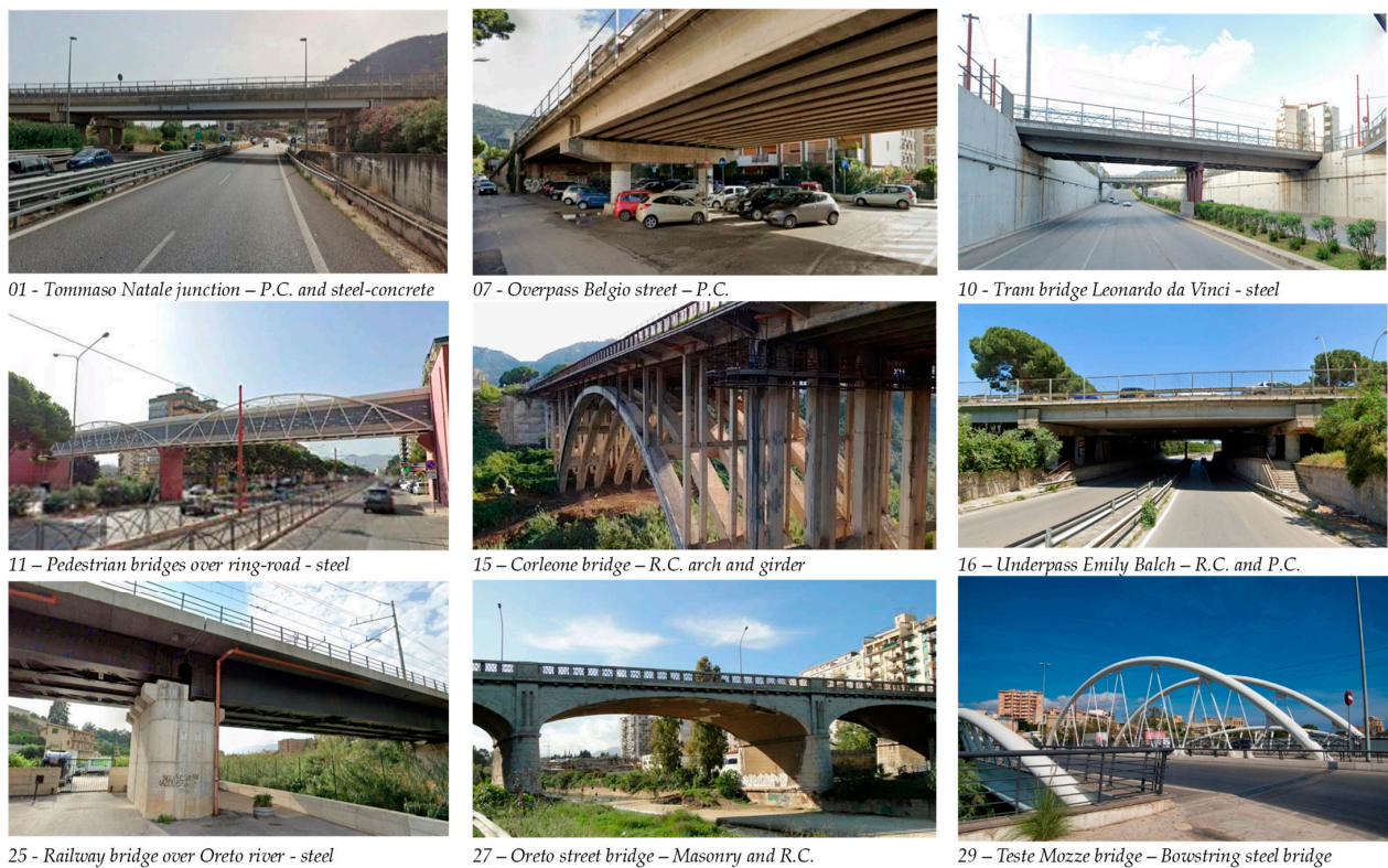
Figure 2. Examples within the stock of bridges considered for testing the procedure of risk-assessment in urban areas.
