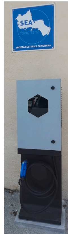
Fig. 2. AME V2G charging point, operated by SEA S.p.A. (DSO in Favignana) and installed in Favignana as part of the BLORIN project.
