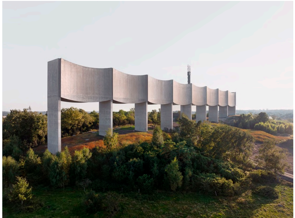
Figure 12. White Arkitekter's Våga water tower in Varberg, Sweden, is a striking 187 m-long (614 ft) concrete structure designed to supply drinking water to nearby villages while serving as an architectural landmark. © Joacim Winqvist, Anna Kristinsdóttir, 2024.
