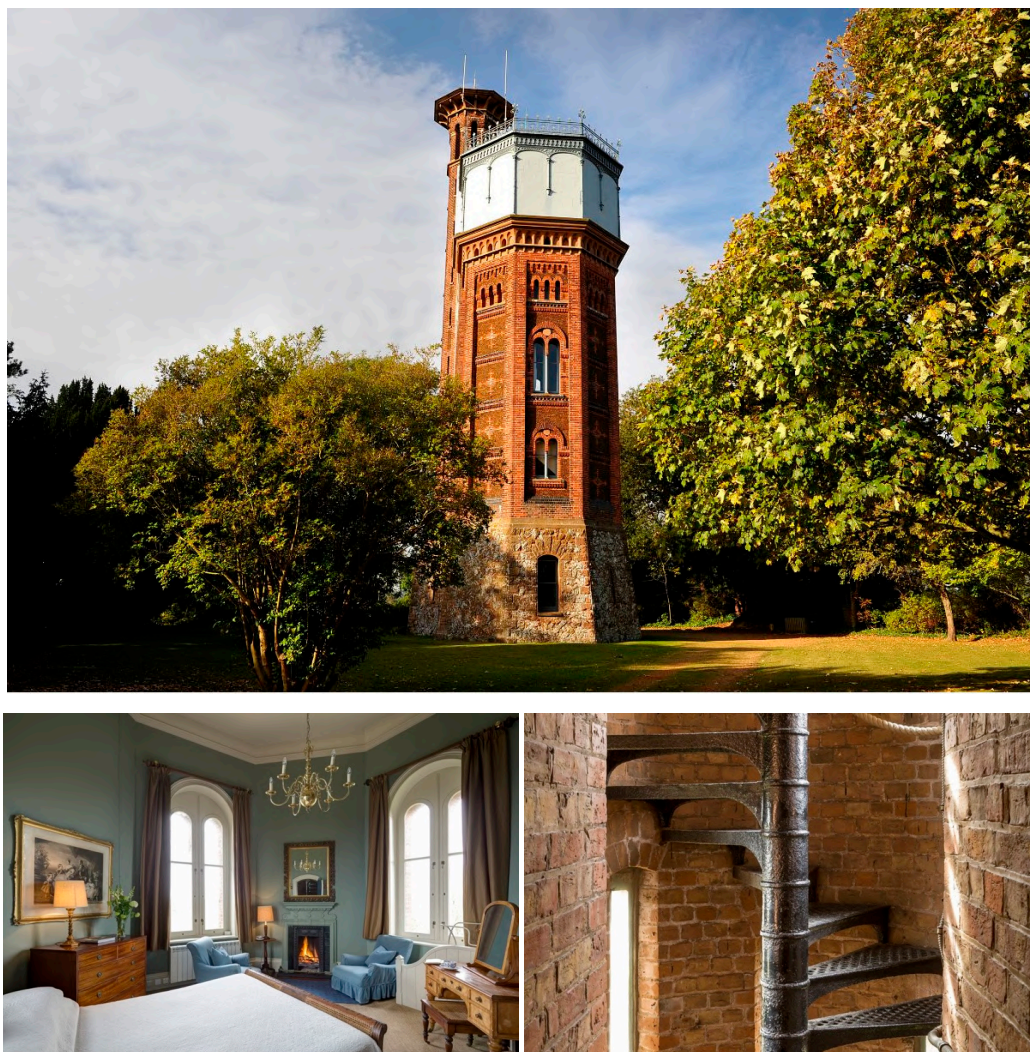
Figure 15. Appleton Water Tower; © The Landmark Trust, 2025.
