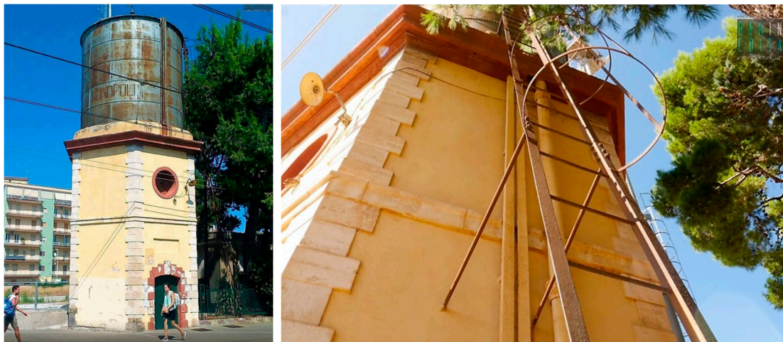
Figure 13. Water tower at Monopoli Railway Station; © Bari Inedita, 2016.
