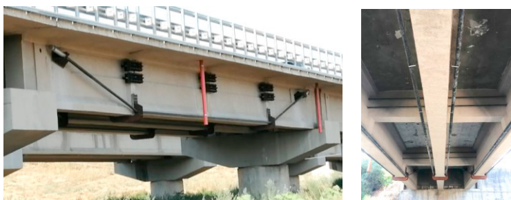
Fig. 5 Example of bridges strengthened by external prestressing.
