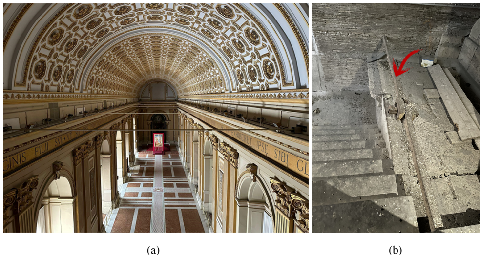
Figure IV.17: Structural tie-rod systems in St. Peter's Basilica: (a) a tie-rod system at the vault springing level of the Hall of Blessings (placed in 1999), and (b) ancient tie-rods inside the north tower.
