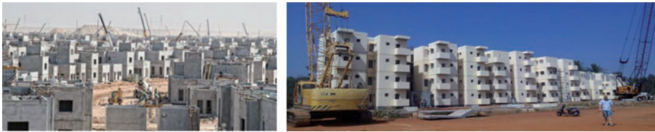
Figure 14. On left & right, illustrate housing compounds constructed with precast concrete. (Zuhairi bin Abdel Hamid).
