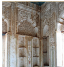
Figure 42. A detailed corner of the wall slots inside the Hussein Rifai house.
