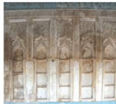
Figure 43. Wall slots inside the Hussein Rifai house.
