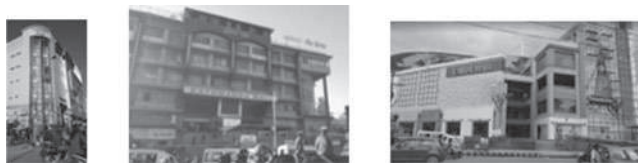
Figure 6. New commercial built forms in the major commercial hub of Kathmandu (Sources: (left, middle) Site visits; (right) Retrieved from www.labimmall.blogspot.com ).
