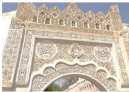
Figure 25. Front façade of the sitting hall of the Ahmed Munawar Al Rifa'i house (AD 1922).
