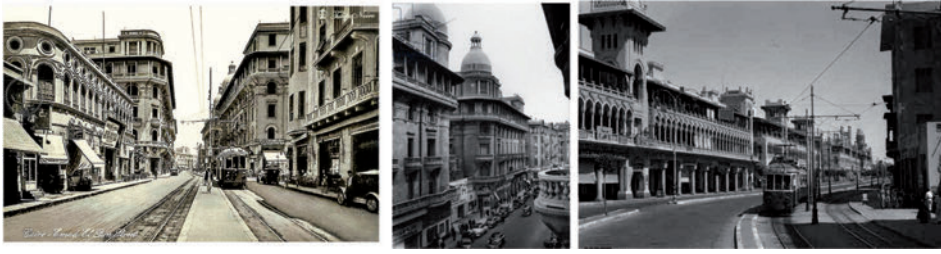
Figure 3. (a) on left and middle illustrate the heart of Cairo in Egypt. ( https://i.pinimg.com/ , 2006) ( https://i.pinimg.com/ , Old Cairo, 2006) – (b) on right illustrates Heliopolis design in the beginning of 20th century ( http://www.egy.com/ , 2008).
