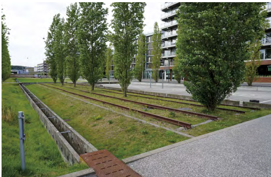
Figure 6.5 Water Retention Basins in Godsbanearealet. ㄱ
