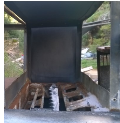
Particular 3. 2 nd Switchgear
