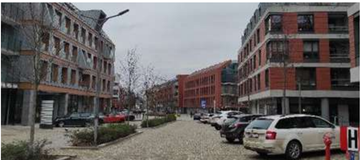
Fig. 6. Housing Projects near the Leibhusaren-Kaserne
