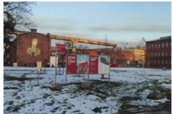
Fig. 8. Directorate building of the shipyard
