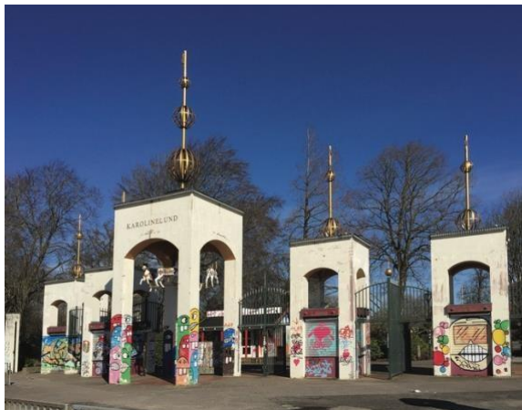
Fig. 10: Entrance pavilions to the disused amusement park of Karolinelund.
