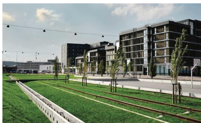
Fig. 15: Rainwater collection and channeling system in Godsbanearialet.
