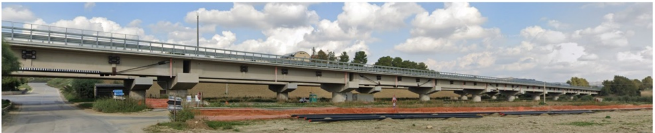
FIGURE 1 | Panoramic photographic view of the multi-span concrete viaduct.
