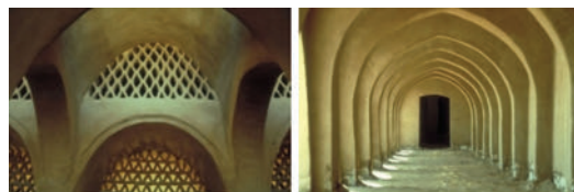
Figure 2. Architect Hassan Fathy used mud brick as a local construction material in the project New Baris Village, Kharga, Egypt. His design represents an ideal expression for the architectural identity for this particular location. (Archnet, 2014).
