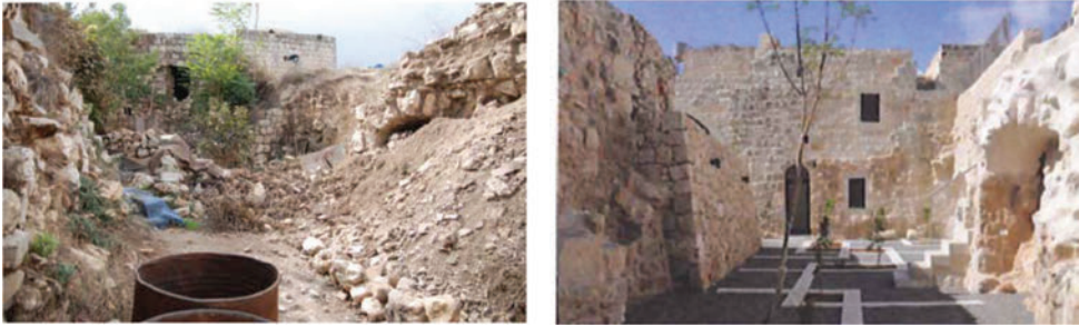
Figure 4. Birzeit Guest House before and after development (Aga Khan Award for Architecture, 2013).
