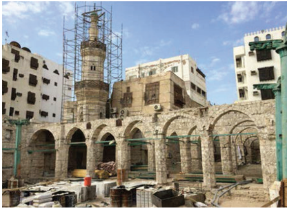
Figure 16. Restoration of Al Shafee' mosque.
