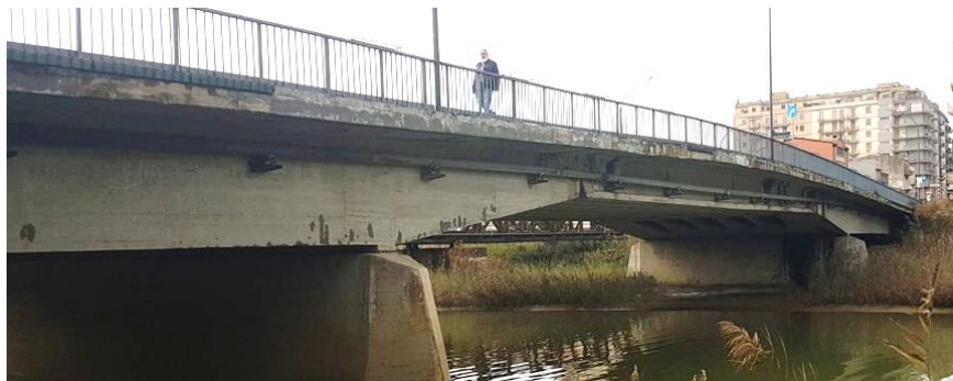
Fig. 4 View of the bridge.
