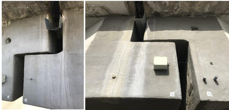
Figure 17. Concrete jacketing of Gerber saddle with CFRP fabrics.
