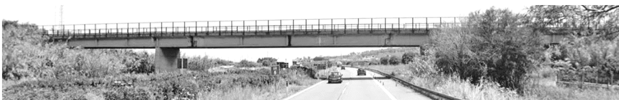
Figure 11. View of the overpass.
