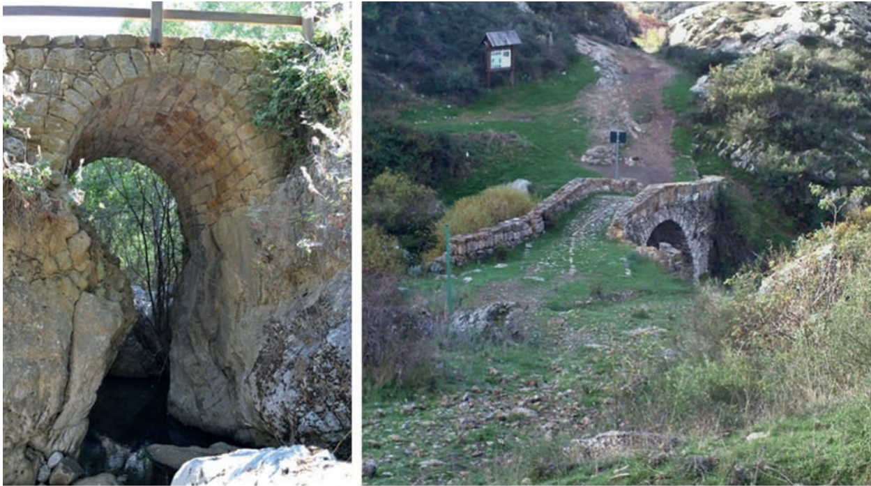
Figure 6 – Sant'Elia bridge (left) and San Pancrazio bridge (right)
