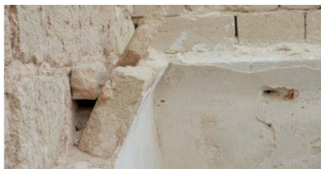
Fig. 15. 'Realina' tiled vault spring (Source: Mami, 2018)
