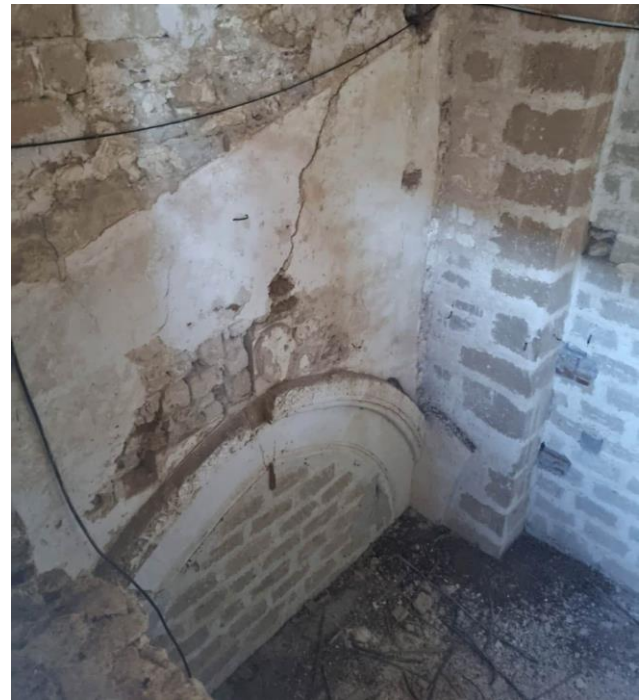
Fig. 8: View of the eastern wall of the presumed dismissed transept: remnants of the pointed arch of the lateral chapel.
