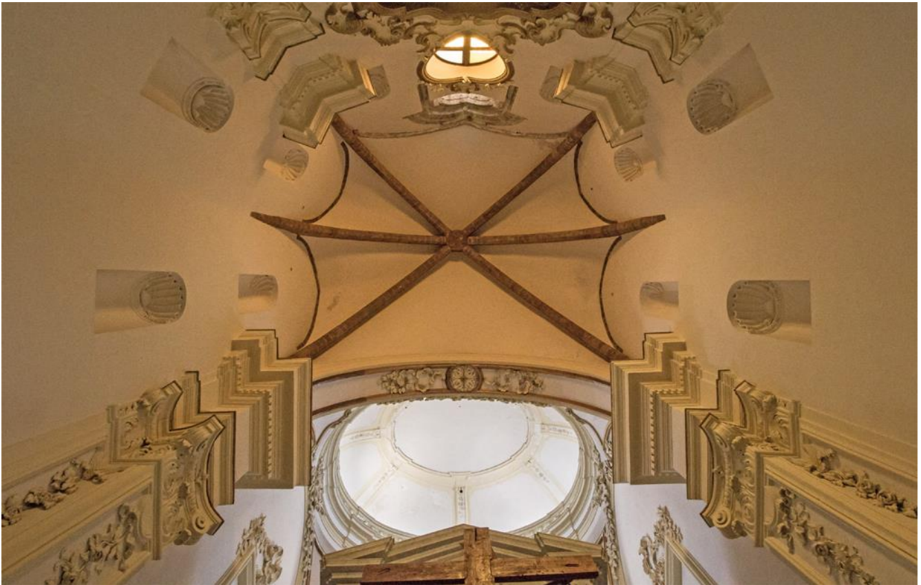
Fig. 2: View of the dome and main gothic apse
