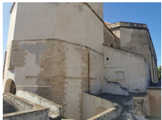
Fig. 6: View of the main apse and presumed transept (north).
